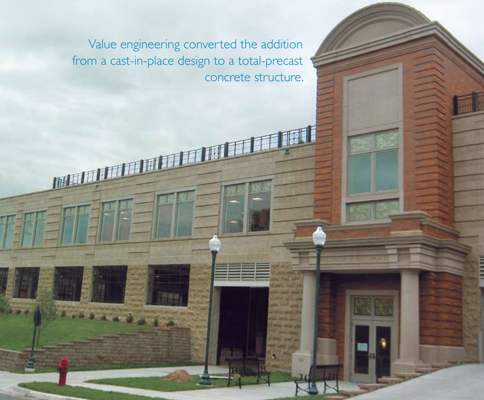
The new entrance to the Stillwater Library is located in the new addition, which features precast concrete panels that replicate the look of the original building.
